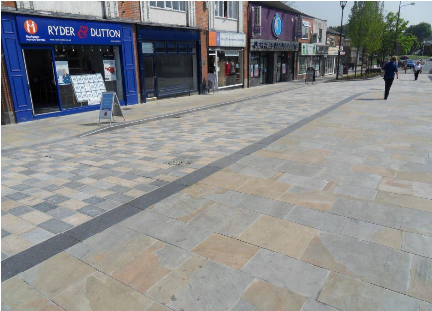
Above: Granite channel and setts to servicing areas
